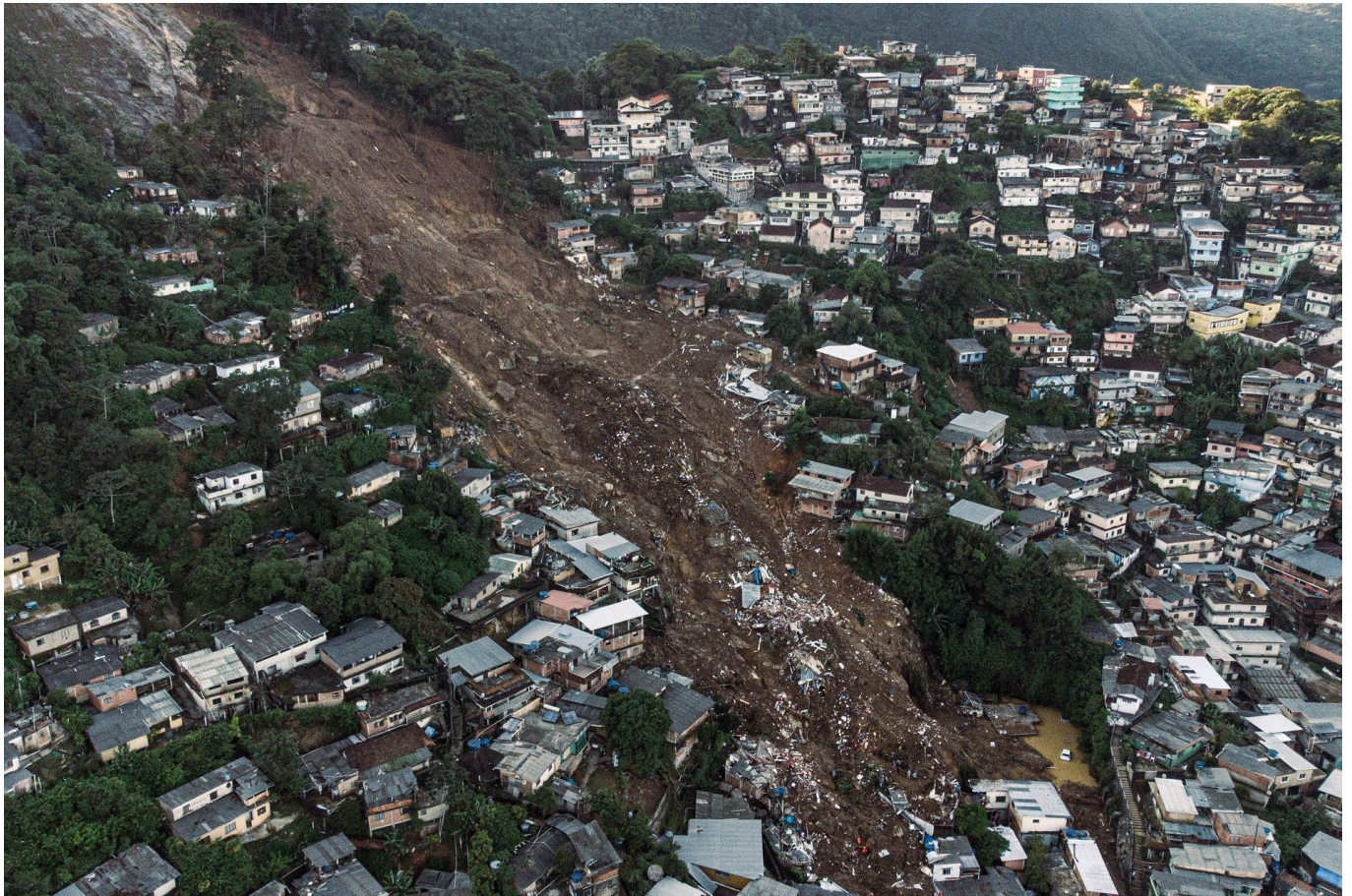
Figure 8: Landslide in Alto da Serra, Petrópolis, where 300 died. Source: National Geographic.
