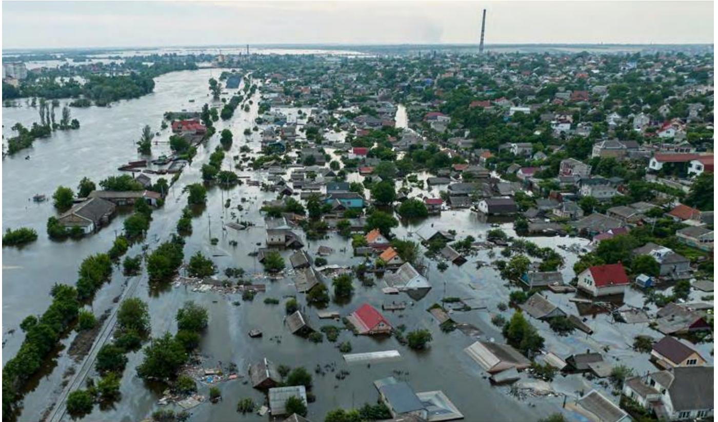
Figure 2: Flooding of the Dnipro River after the Kakhovka Dam breach. Keystone/AP.
