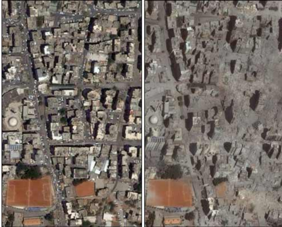
Figure 2: Harat Hurayk quarter of south Beirut before and after the Israeli bombings. Source: Digital Globe
